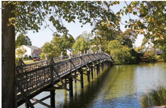
Footbridge over Spring Lake
